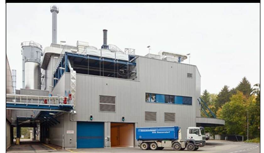
Sewerage-sludge incineration plants
